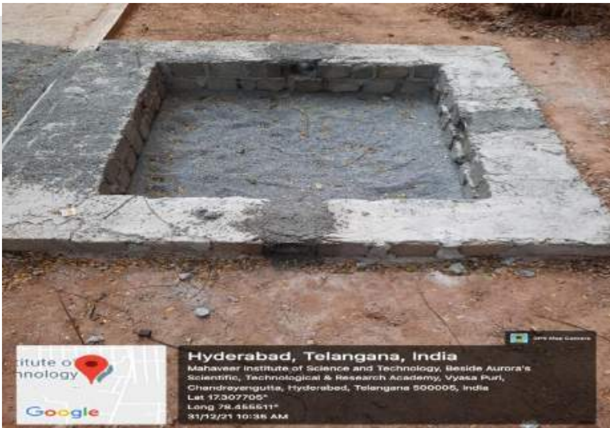
RAIN WATER HARVESTING PIT
