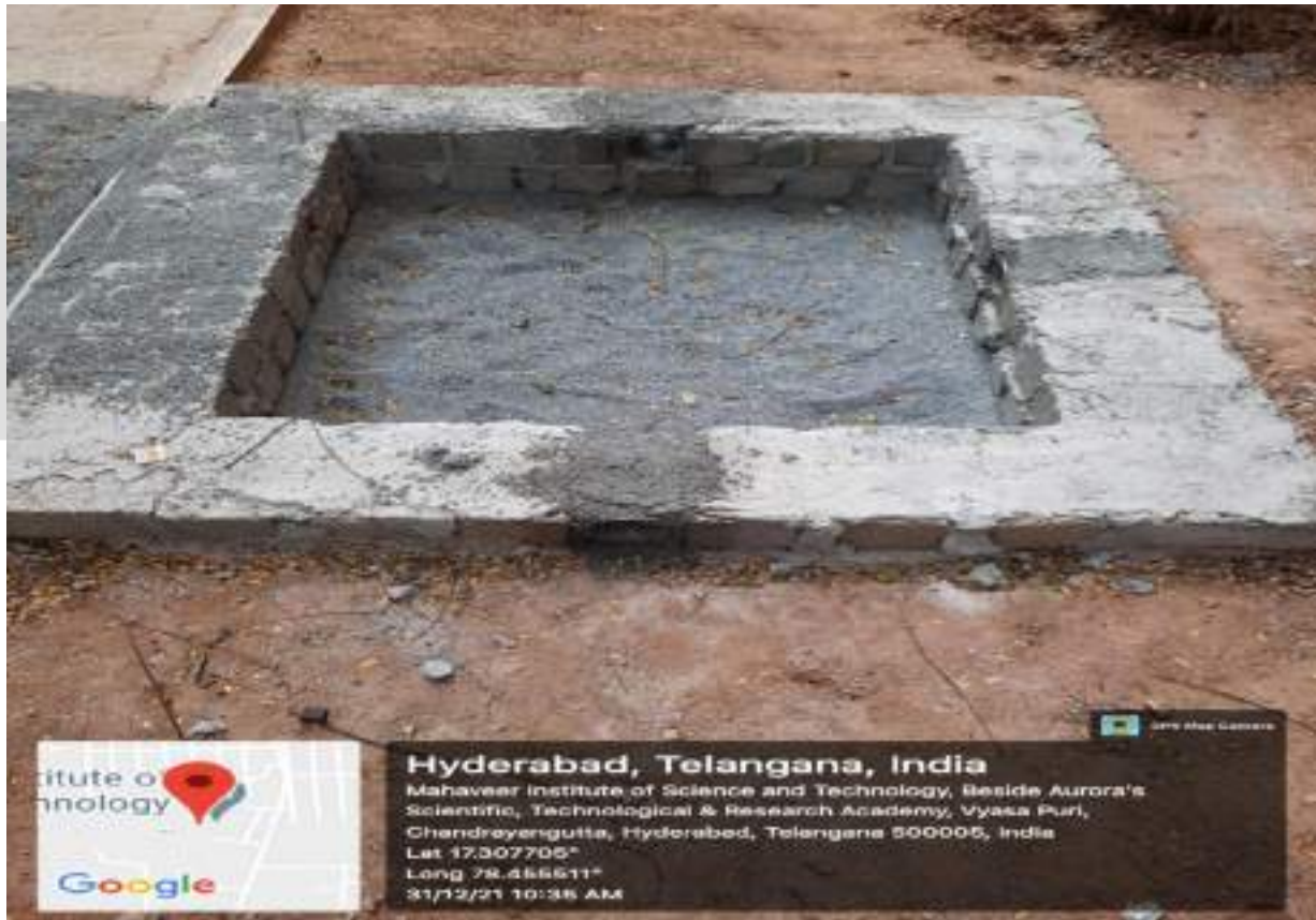
RAIN WATER HARVESTING PIT
