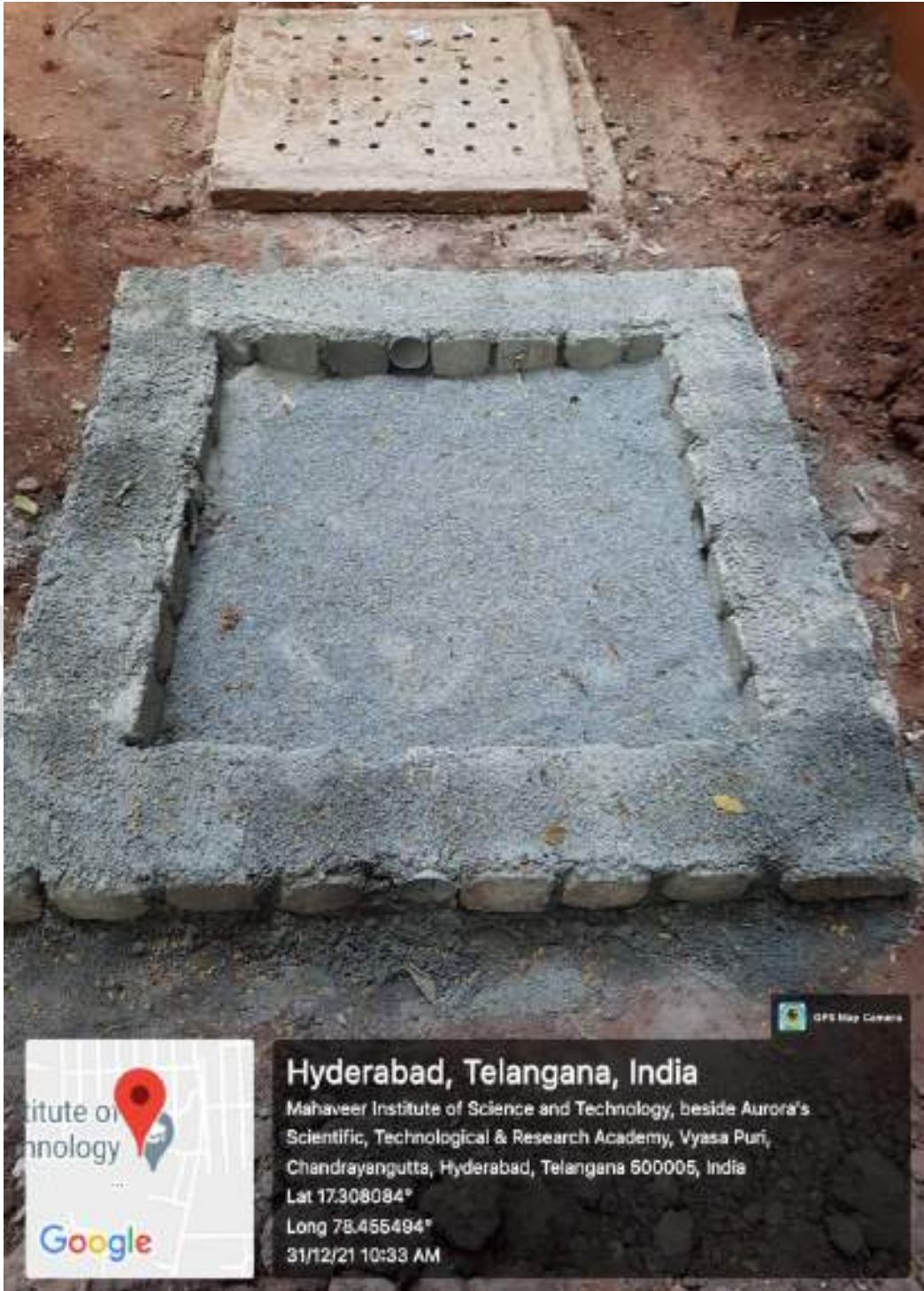
RAIN WATER HARVESTING PIT
