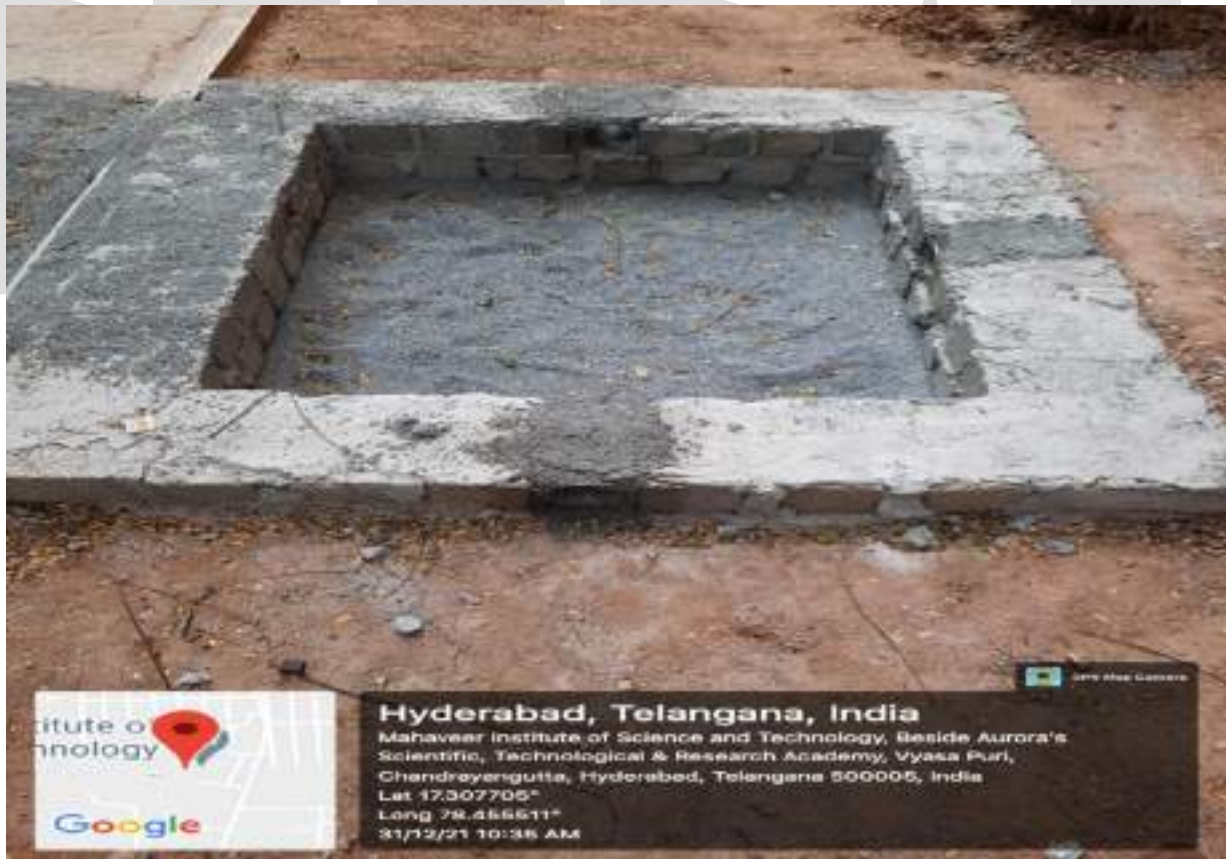
RAIN WATER HARVESTING PIT
